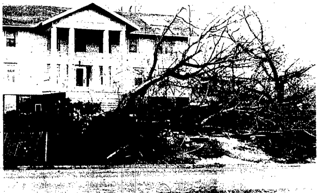
Preparation for expansion of the Wayne Retirement Center began Thursday with the clearing of trees from the property. Owen K. Dahl said construction would be in three phases, the building of a two-story section in front of the old Lutgen Hospital; the tearing down of the old building, which was converted to a nursing home in 1948; and the construction of another two-story unit where the old building now stands, with a courtyard and corridor connecting the two new units. The 18,400-square-foot addition is expected to be completed by the middle of December. Ofte Construction Co. of Wayne has the contract.
